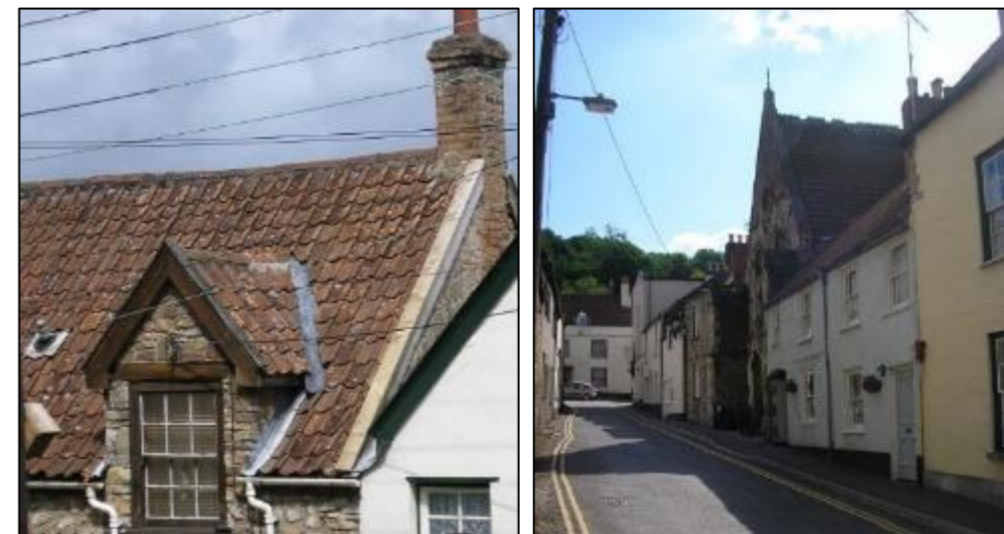
Figure 8: Examples of roofing materials
