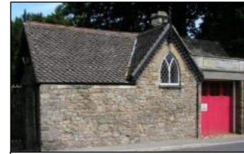
Old Fire Station
