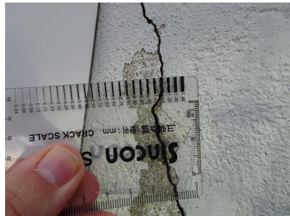
Photo: 2 Crack gauge
